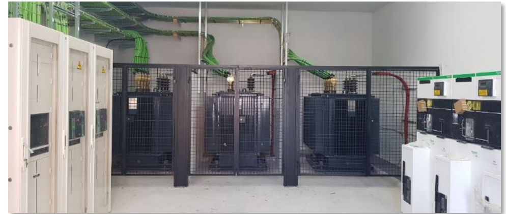
i.e. The new Fuencarral bus depot transformation centre will supply 50 chargers of 80KW
